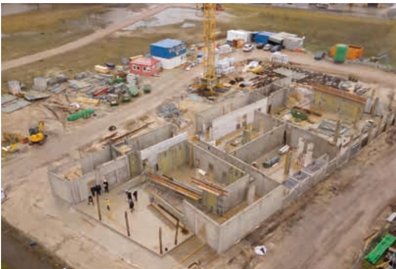
Film shooting on the construction site
